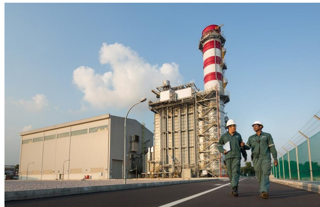
Sembcorp Cogen @ Banyan
