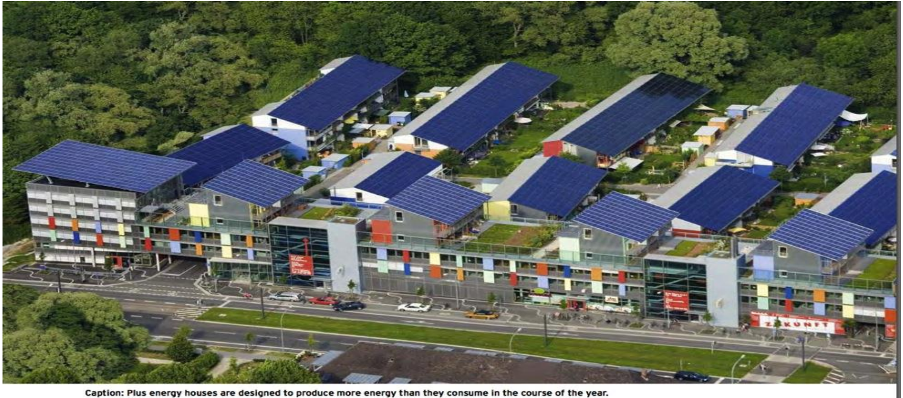
Caption: Plus energy houses are designed to produce more energy than they consume in the course of the year.
